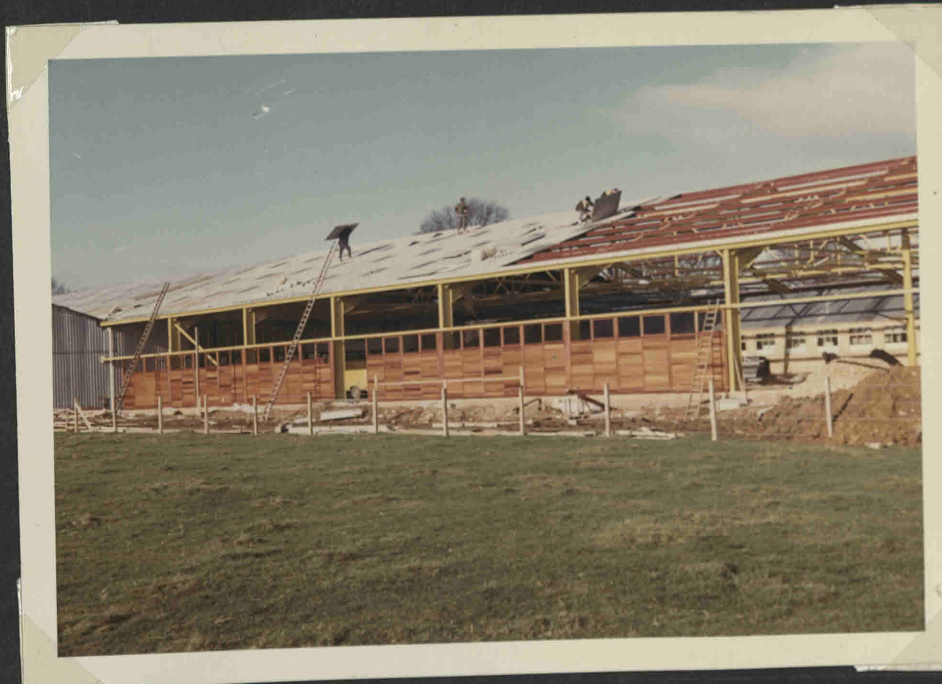
Stages in erection of the extension taken over by P.K. 1st MAY 1968
